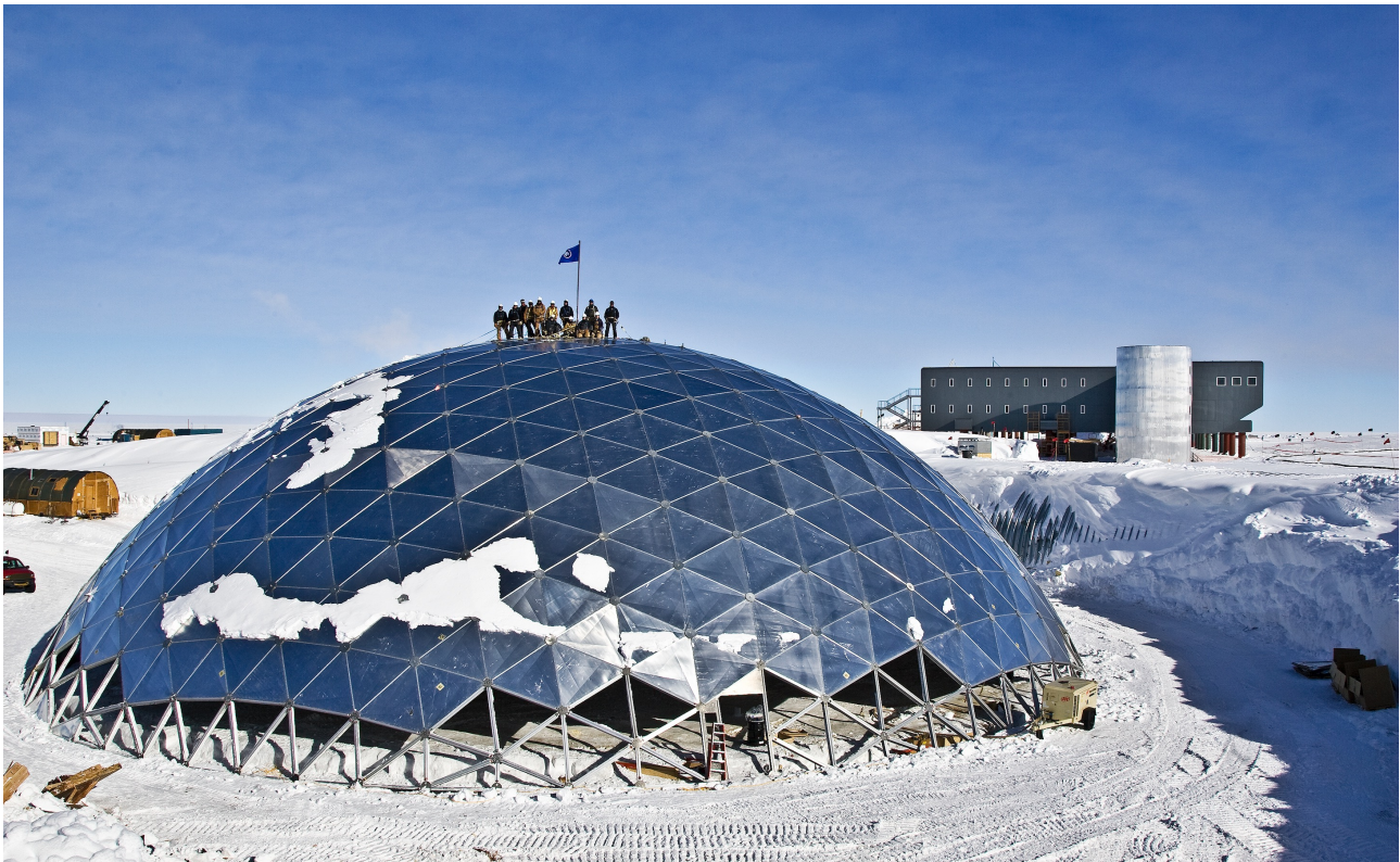
The South Pole Station Dome (being deconstructed)
